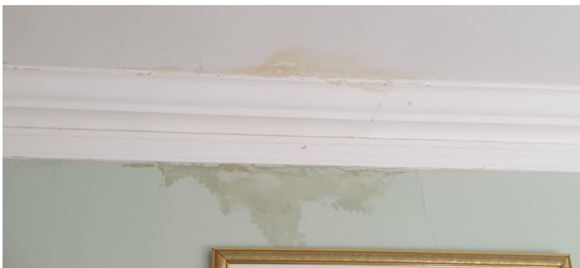
Figure 5: Water damage at 2F, 10 Randolph Crescent due to leaking roof.
